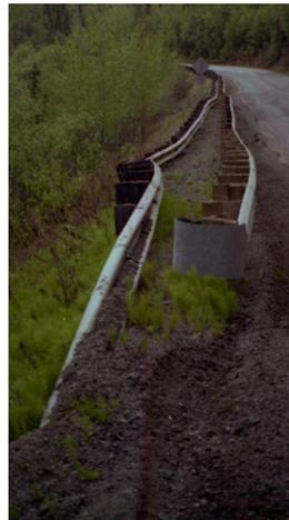
Top of W-Beam guardrail less than 26 - 1/2" when spliced at post only (2017 and earlier installations.)
