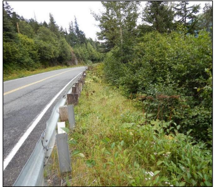
Left: Glenn Highway – Guardrail deflection and post separation
