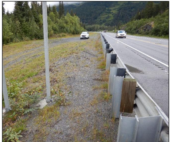
Left: Glenn Highway – Post separation and guardrail deflection
